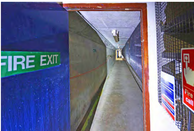
Looking along the Gallery tunnel from the west end
